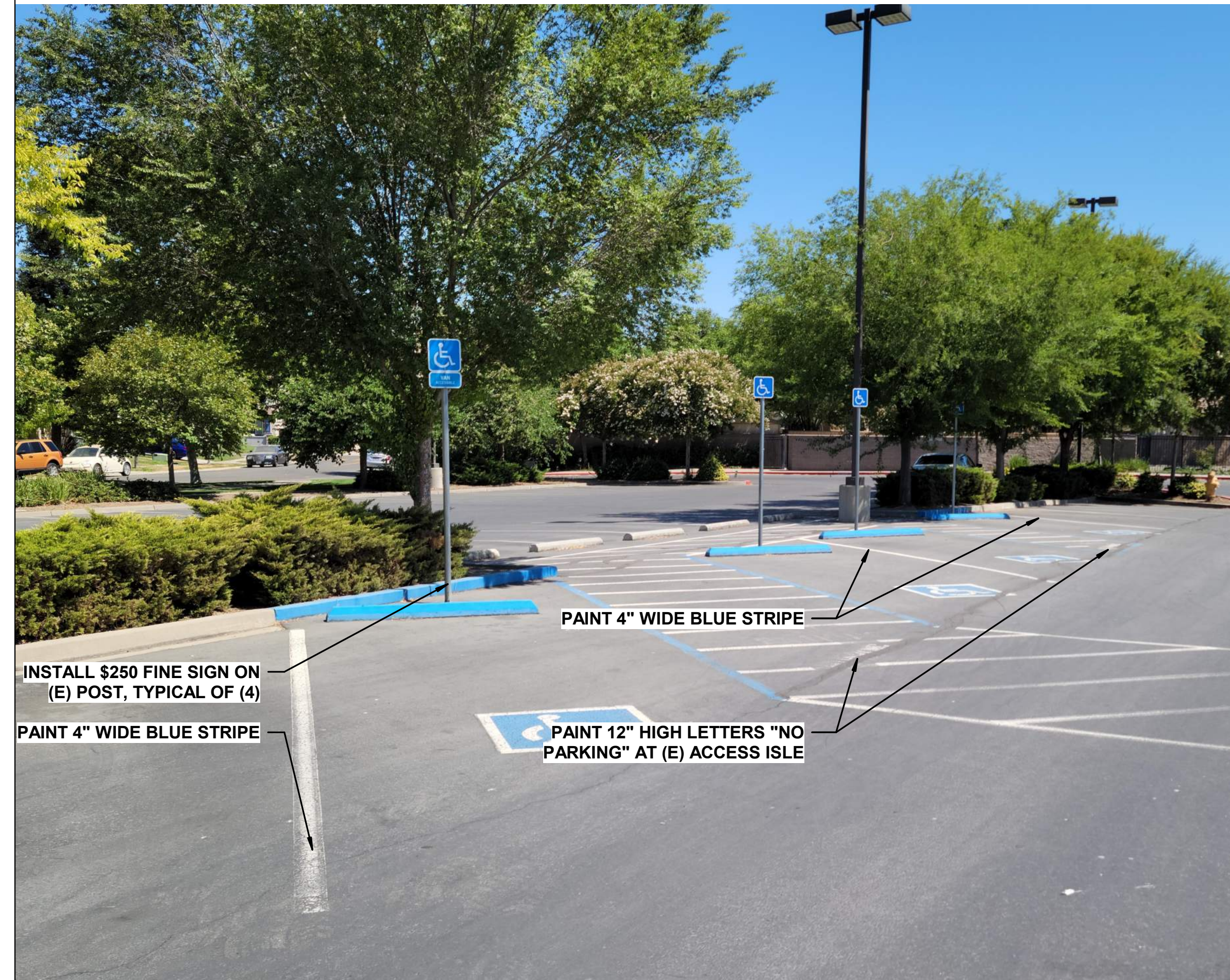
EXISTING ACCESSIBLE PARKING
